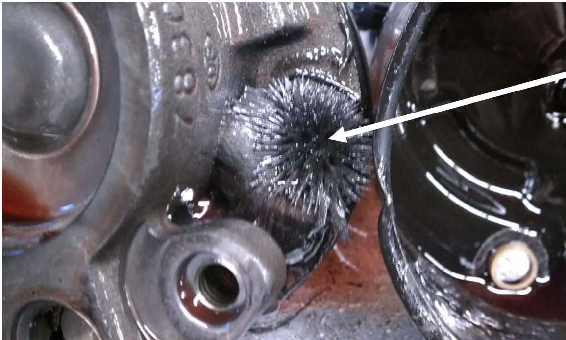
Metal from old System on Magnet
